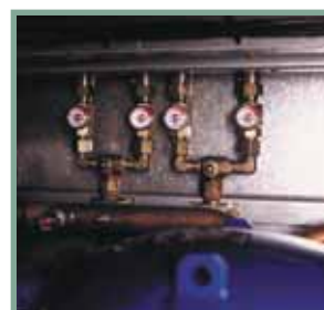
Dual pressure relief valve
